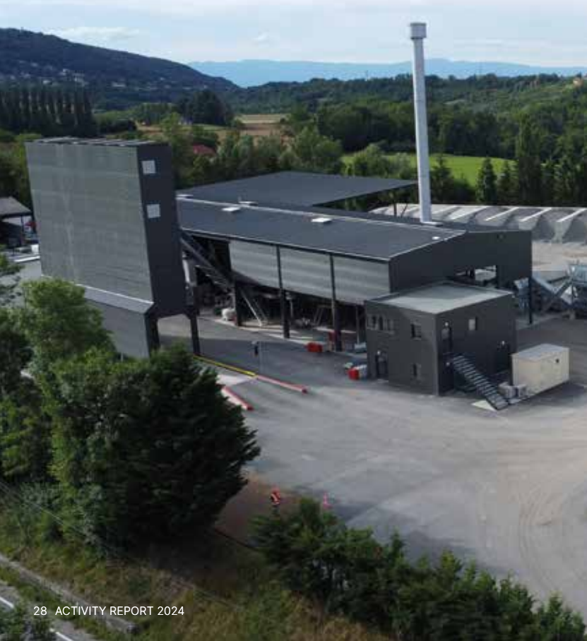
TSX23 INCITY, asphalt plant – Ermont
